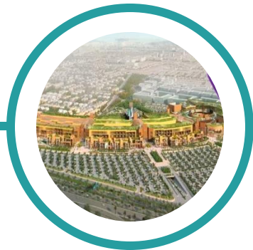
RIYADH Underway (April 2026 opening)
